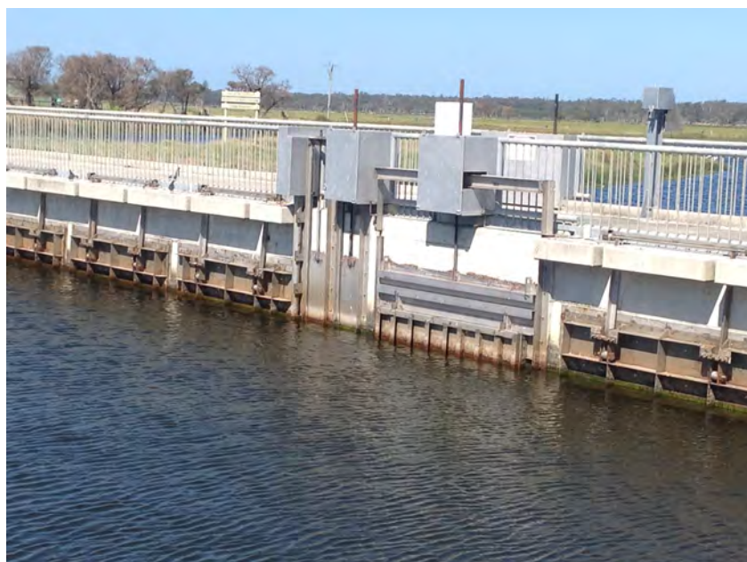
Photo – Wonnerup floodgates (Nov 2013)
