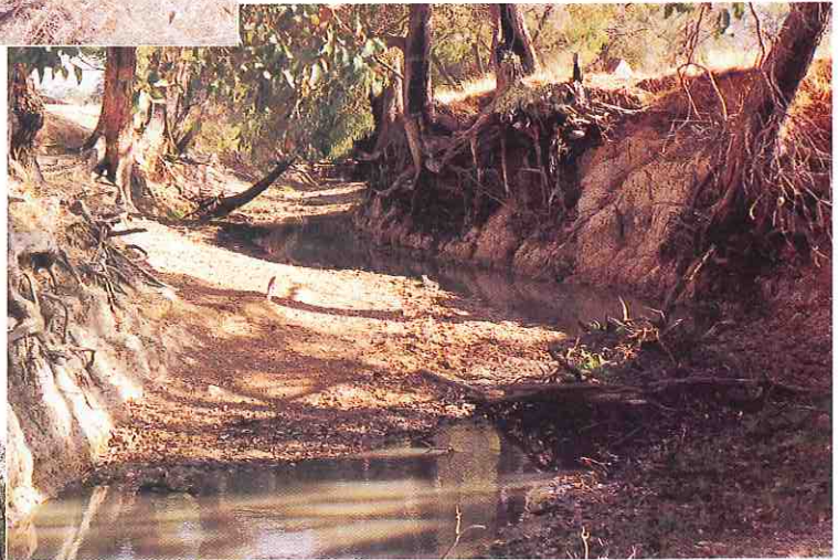
C3 foreshore on the Sabina River. Soil is being washed away from between tree roots and the undermined trees are at risk of falling into the river. This will cause ongoing erosion problems.
