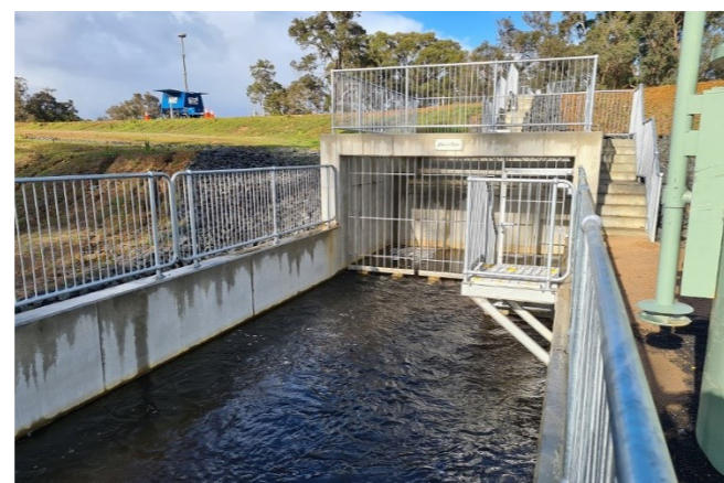
The completed penstocks
