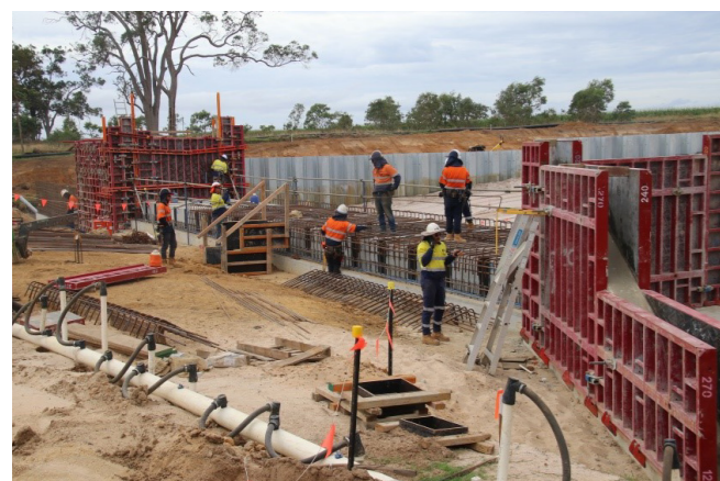
Installation of the culverts and penstock
