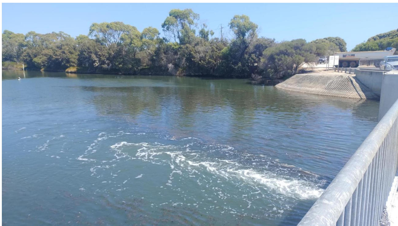
Photo: seawater in-flow to the Vasse Estuary in March 2025.
